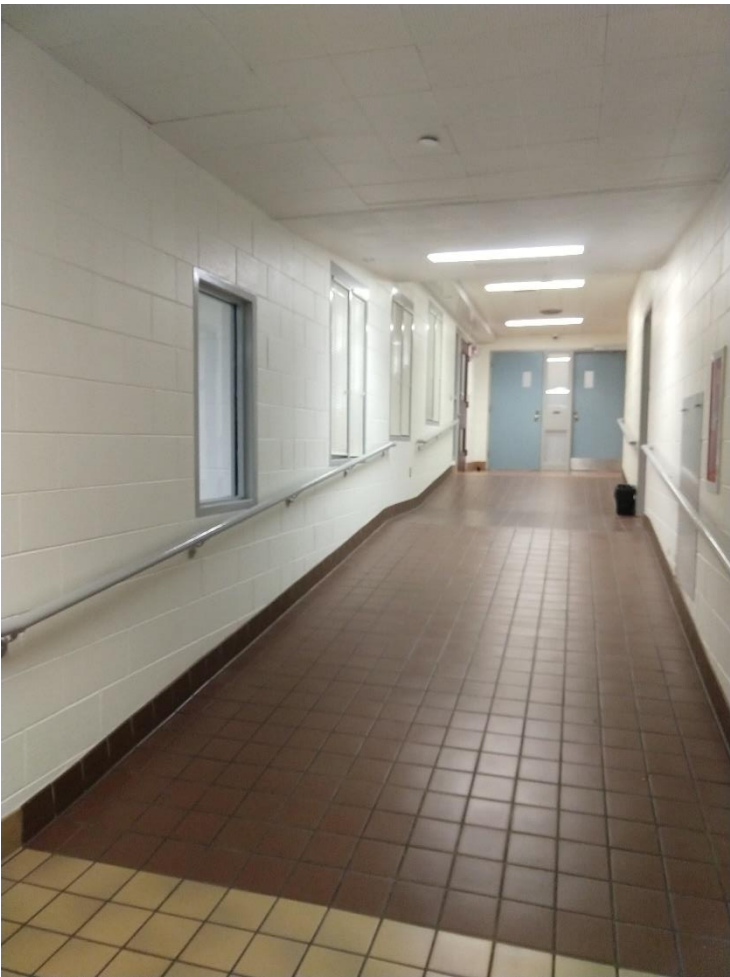
Ramps Through-Out Jail
